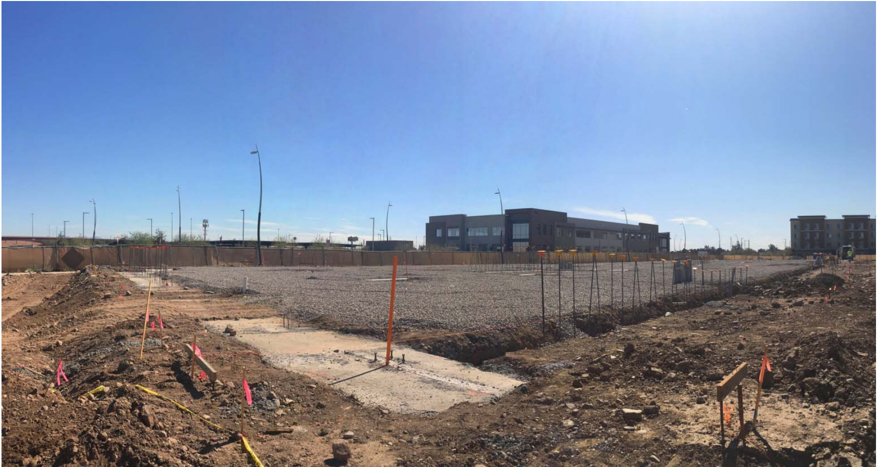
Vapor Mitigation System Installation Completion Rio Salado Pkwy, Tempe, AZ
