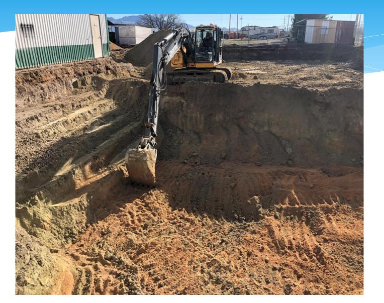
Even with today's rapid turn-around timeframes for analytical results, excavation zones may be open for (2) two to (5) five days before post-remediation cleanup verification analytical results are available. During the interim time, excavations may be left open presenting a physical hazard, or the excavation zone may be backfilled presenting a potential for duplicating work re-excavating due to unanticipated analytical hits.
