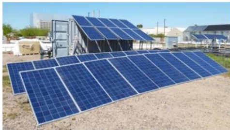
Unpacked and powering 20 kW of loads
